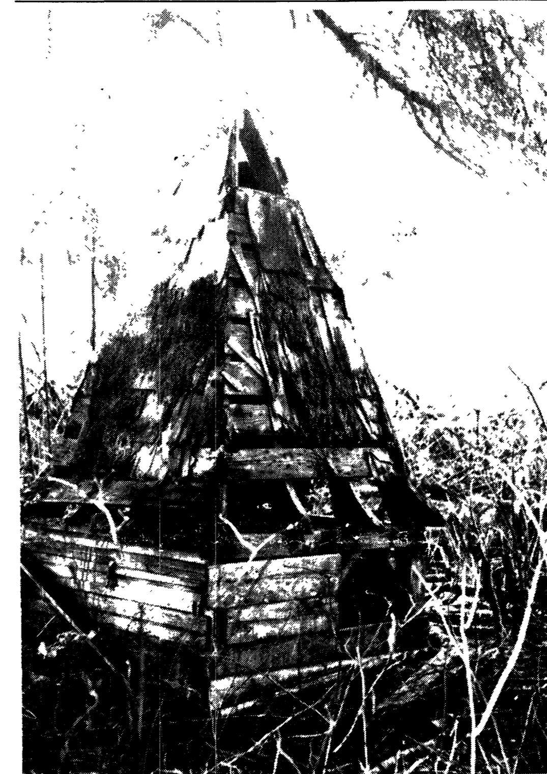
FROM THE PAST--A few shingles still cling to this weathered structure which once served as a steeple for the old Quillayute Prairie Church. The church is gone now as are many of the pioneers who worshiped here. Moss has now taken hold and will soon cover this skeleton as it gradually gives way to brush here on the Quillayute. ---Lonnie Archibald
